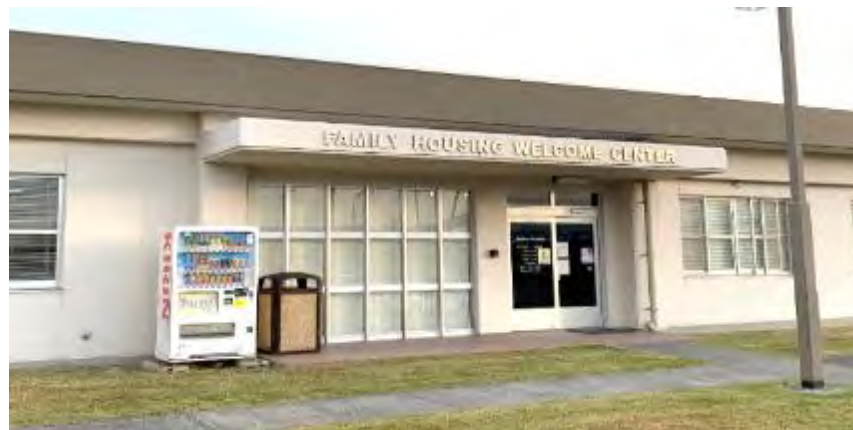
Family Housing & Self Help Building 200
